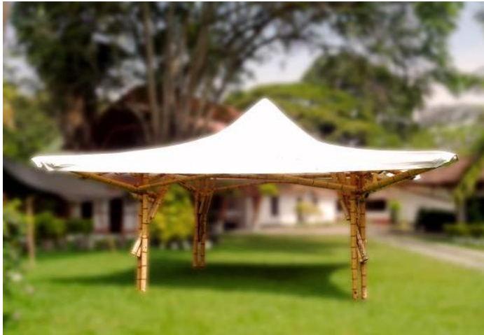
Fig. 5. Modular prefabricated bamboo structure based in linear elements with PVC covering.
