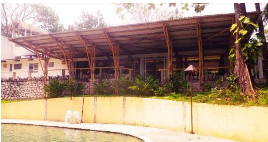
Fig. 2. Planar modules in parallel creating a gallery.
