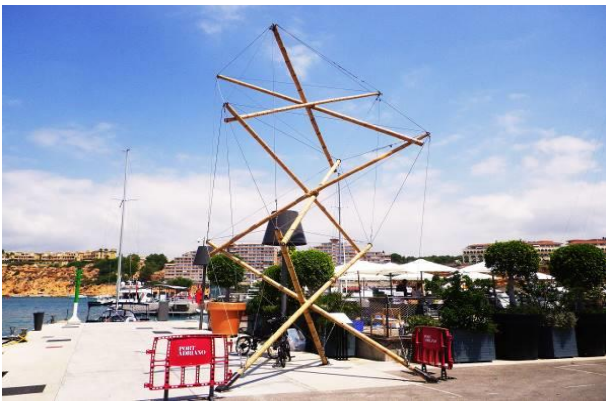
Fig. 3. Spatial modules conforming a 8-meter-high tensegrity tower.
